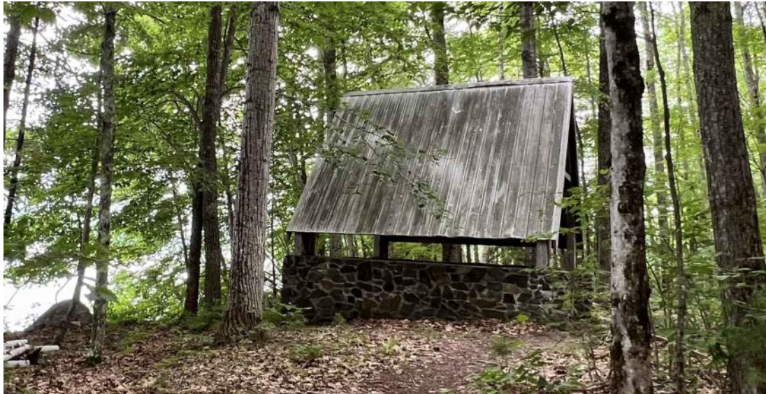
CHAPEL ROOF - BEFORE
