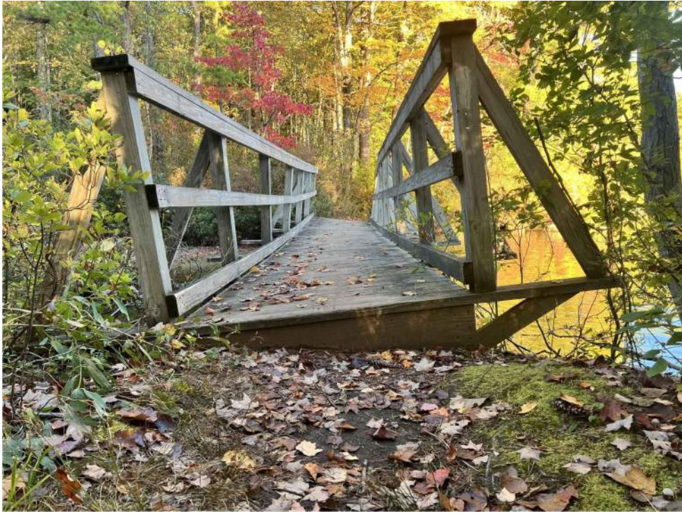
SHORE TRAIL BRIDGE - BEFORE
