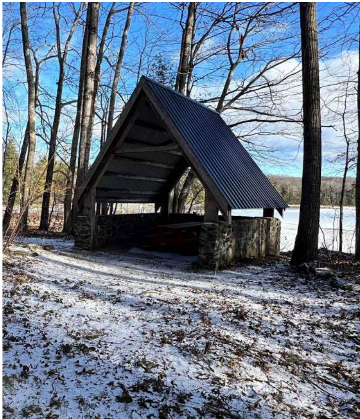
CHAPEL ROOF - AFTER
