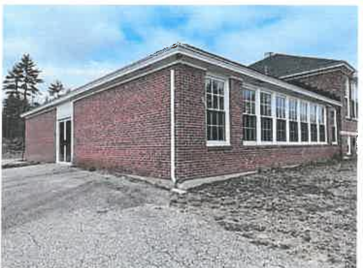
1965 addition on slab
